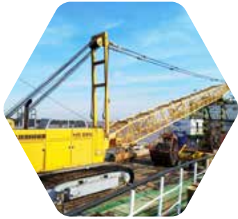
Crawler Crane "LIEBHERR 120 TON"
