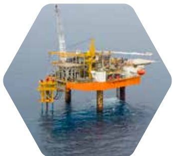
Mobile Offshore Production Unit (MOPU) "MALEO PRODUCER"
