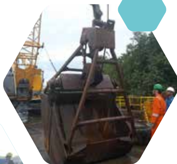
Crane Barge Ex-Package No. 9, East Kalimantan
