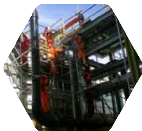
Supporting Booster Compressor Installation, Madura Strait
