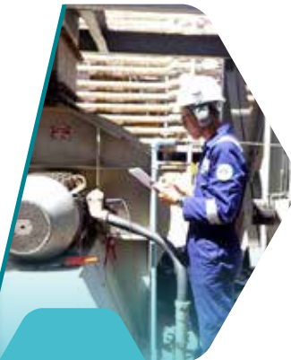
Field Operations Support Services for North Duri Cogen
