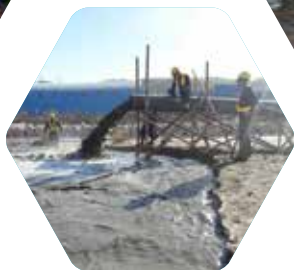
Jetty Dredging Service, East Java
