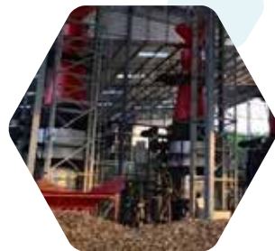
Biomass Power Plant in Nias
