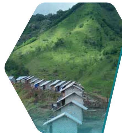
Supply and Installation Solar PV Home System in NTT
