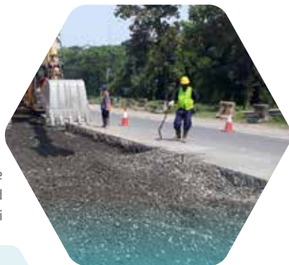
Maintenance Tollroad Jagorawi
